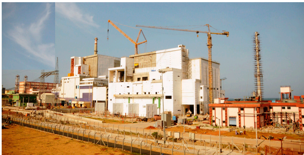
Overall view of Turbine & Nuclear Island Connected Building
